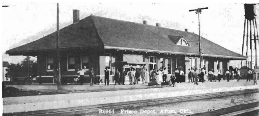
New Passenger Depot, Afton, Okla.
