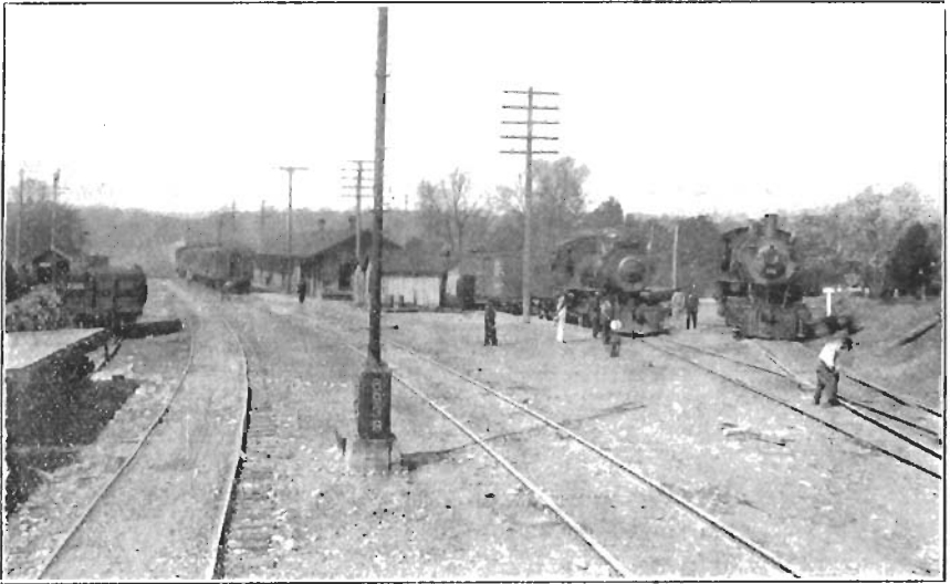
View of yards and station, Jasper, Ala. From left to right may be seen passenger train No. 992, extra 954, switch engine, and I. C. R. R. extra
