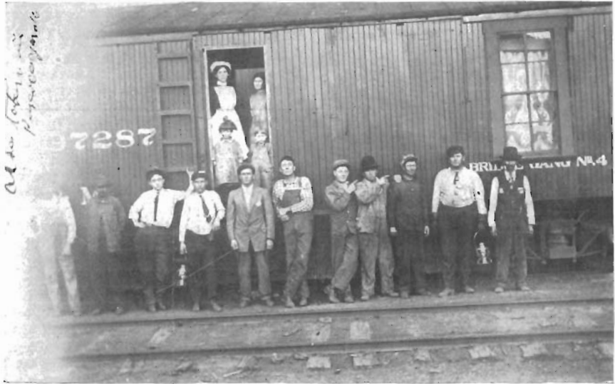
Bridge Gang No. 4, running a small driver on the Hoxie Line. The first man on the right in the picture is
